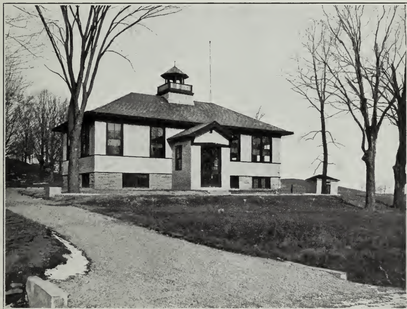
The new building at Fairmont, Onondaga county, School district 3, Camillus
